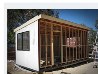
Roof and External Cladding
