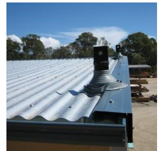
PICTURED ABOVE: Lifting points for site transportation
